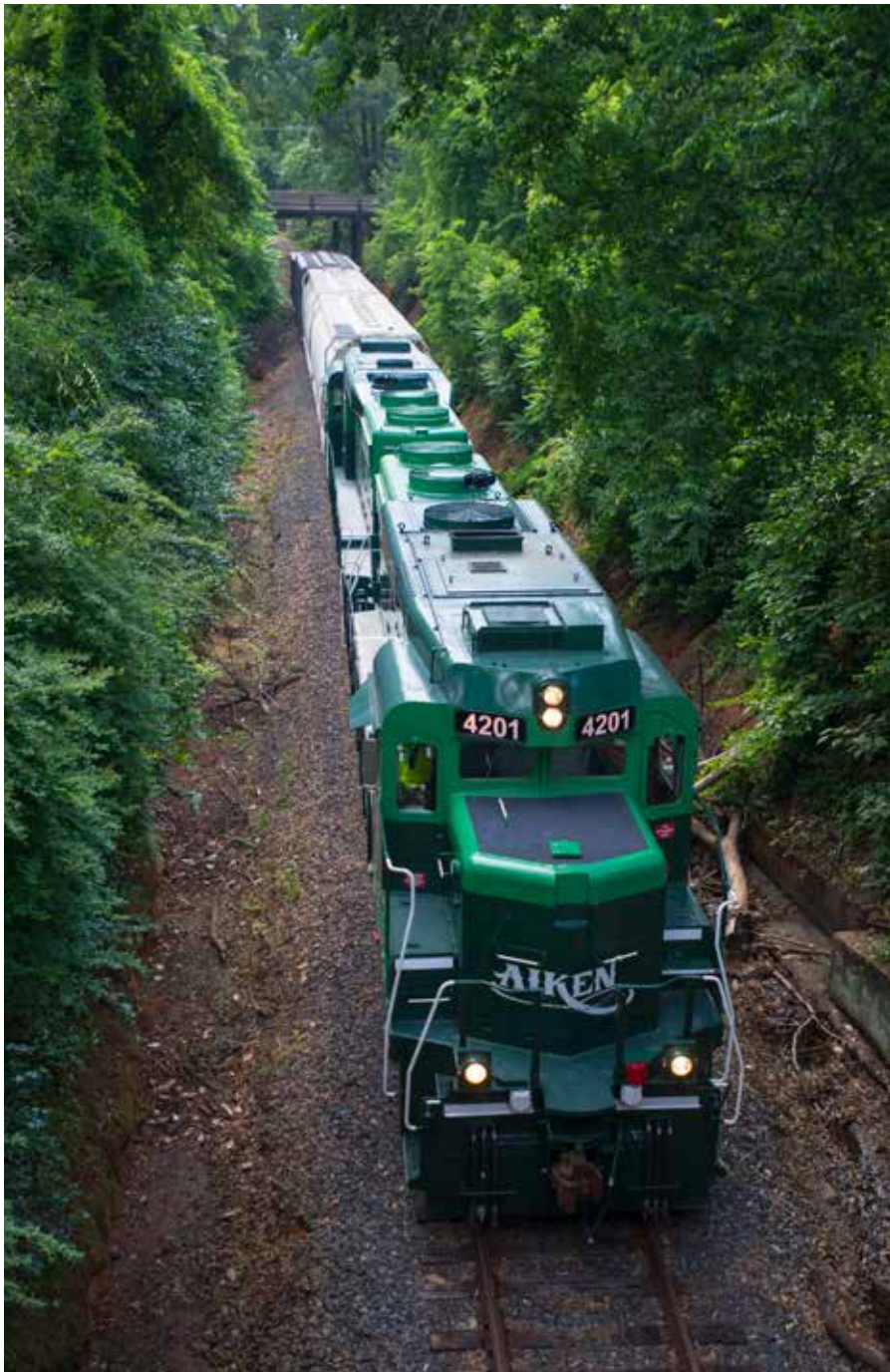
A pair of Aiken Railway GP30s lead a train through the 40-foot-deep cut built in 1852 at Aiken, S.C., that replaced the original incline railway of 1833 to reach this point. Steve Smedley
